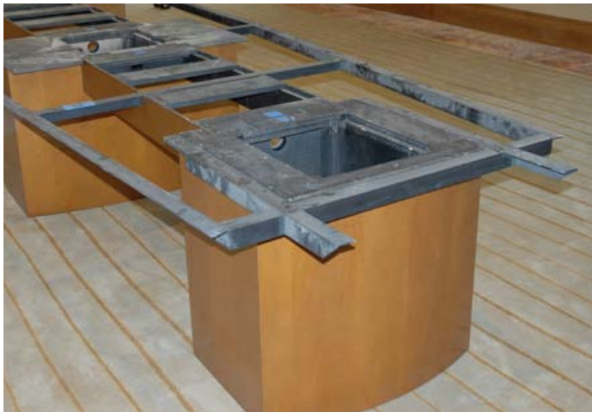
Woodclad steel sub-structure for stone support.
